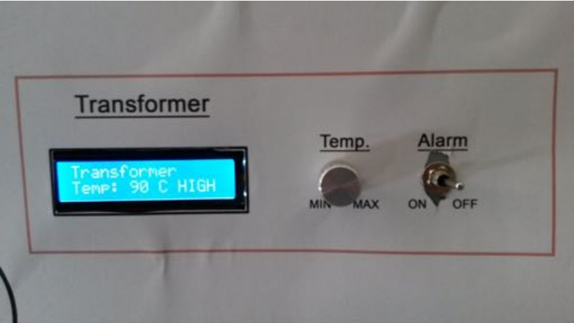
Figure 47, Transformer status, Alarm deactive and HIGH temperature
